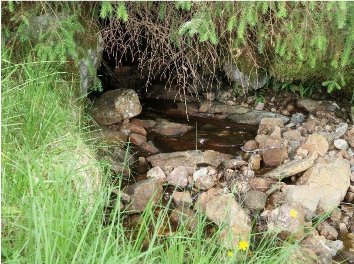
Figure 45: Culvert at the upper end of Transect ACC2.
