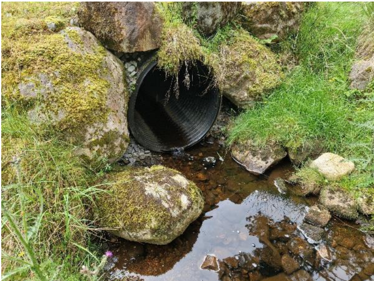
Figure 22: Impassable Culvert (on the day of the survey) at the upper end of the survey stretch.
