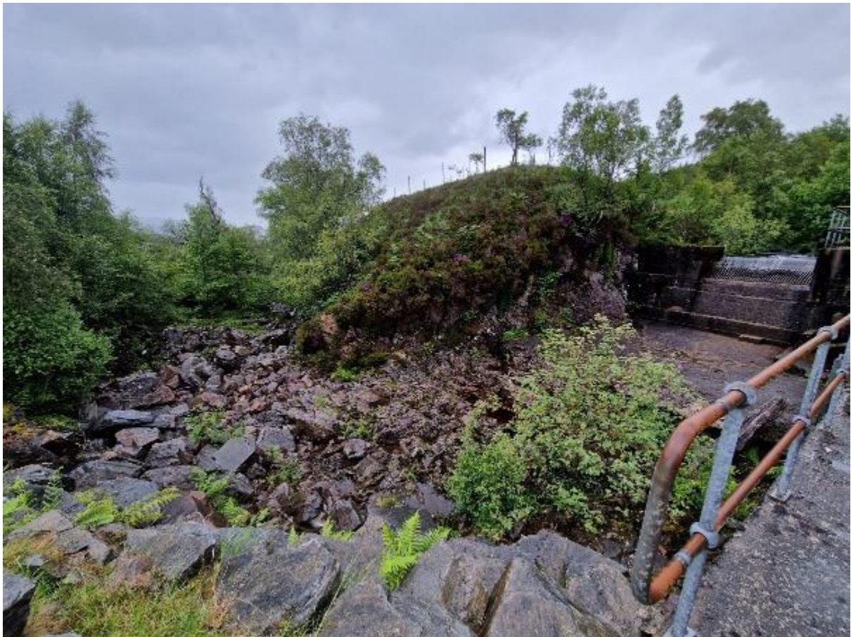
Figure 52: Allt Garbh Doire hydro intake and dewatered section downstream.
