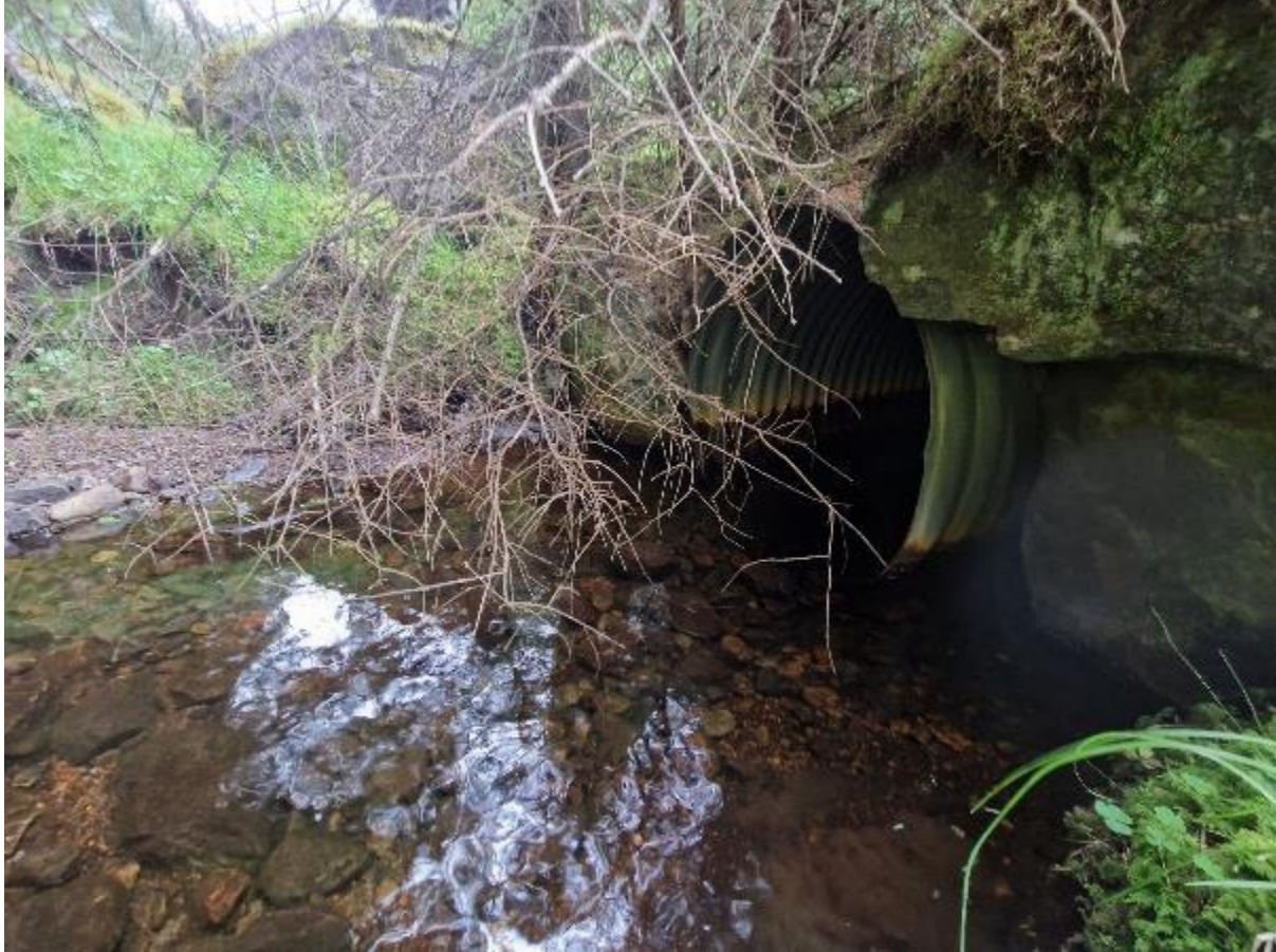
Figure 32: Passable culvert at the upper end of Transect ACB1
